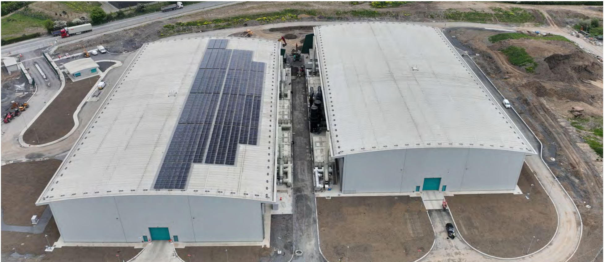
Regional Biosolids Storage Facility during the construction phase
